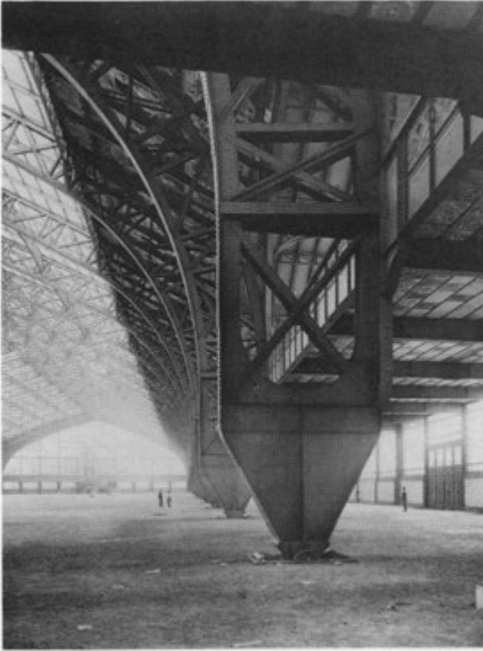
Fig. 40. Paris. World Exhibition: Palais des machines (Dutert and Contamin, 1889)
