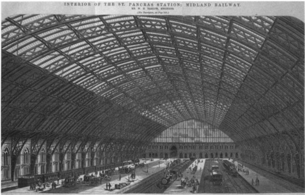
Fig. 39. London. St Pancras Station: train shed (Barlow and Ordish, begun 1863)
